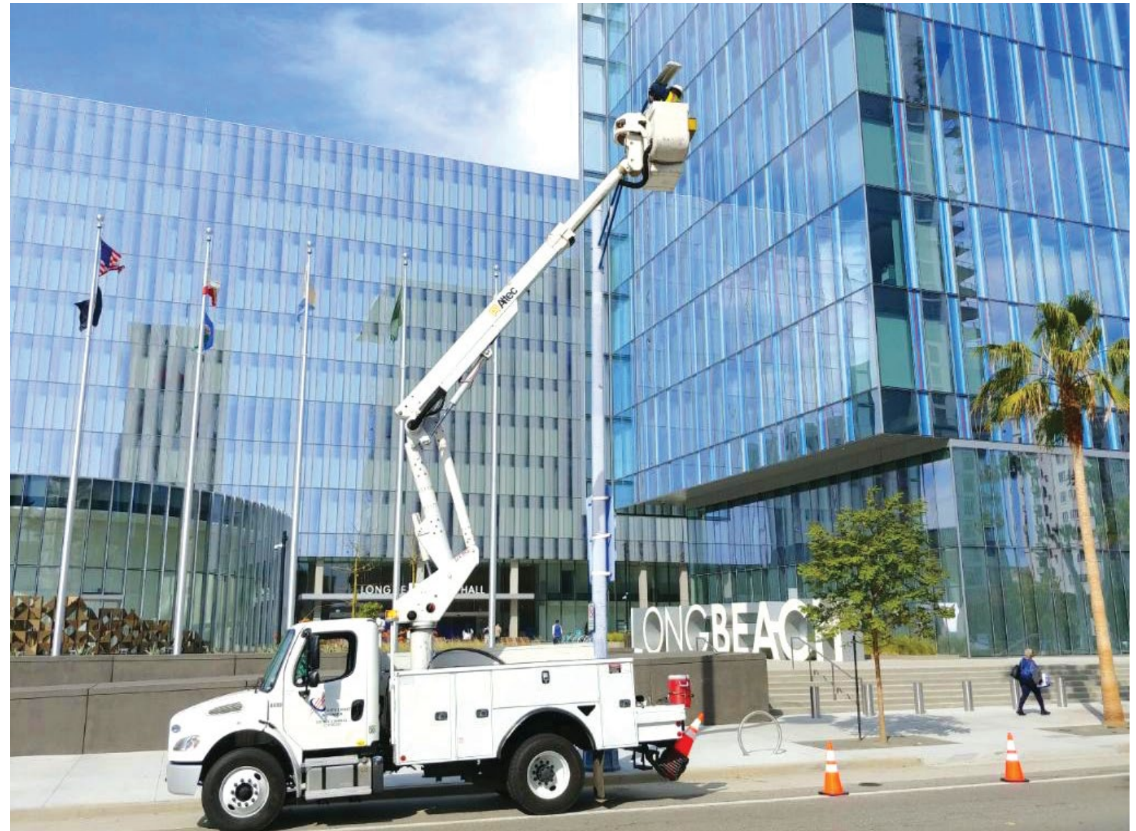
City Light & Power LED Retrofit - Long Beach, California
